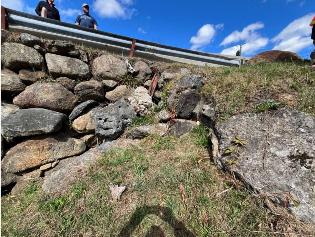
Photo 7: Downstream side of dam at the left abutment contact.
