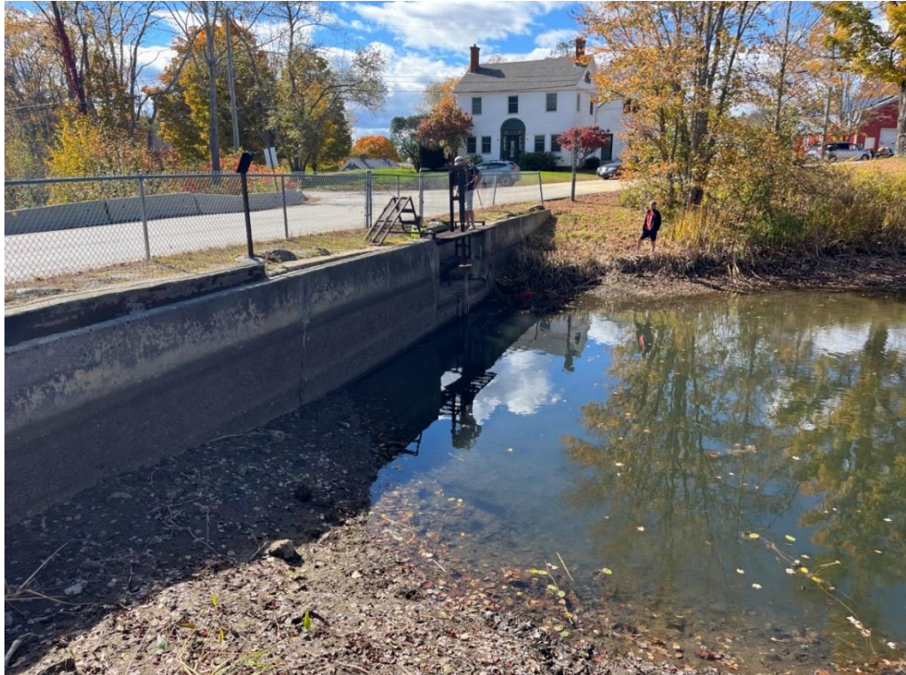
Photo 4: Upstream of the dam from left abutment.
