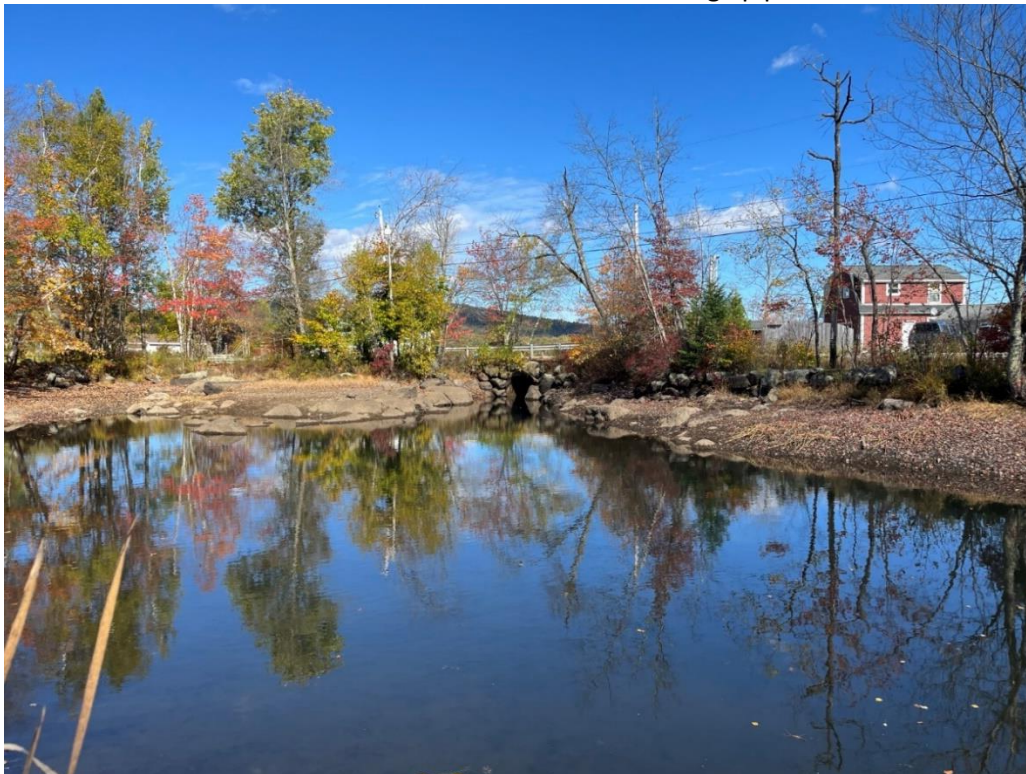
Photo 12: View of pond from top of dam
