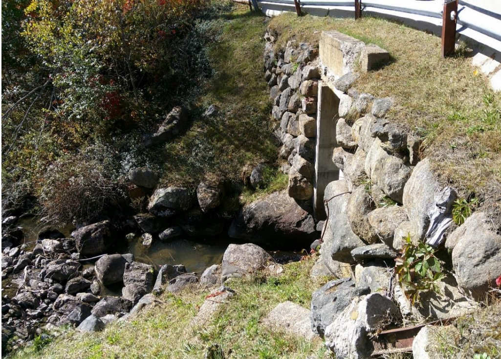
Photo 5: Downstream side of the dam from left embankment.
