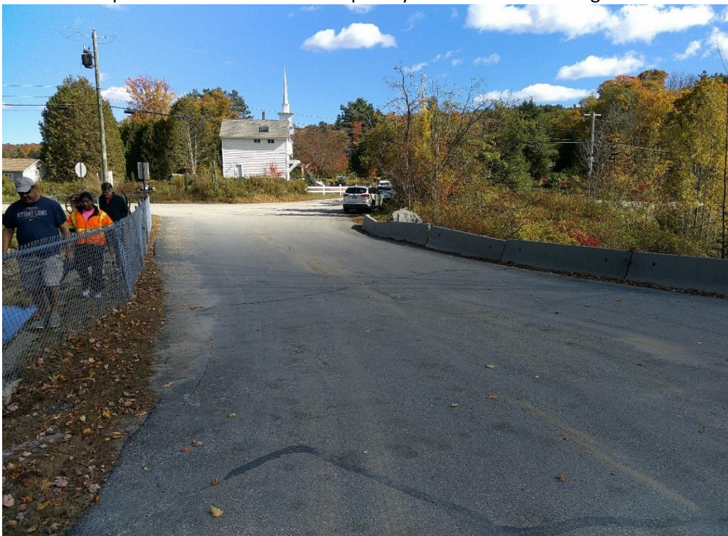
Photo 2: Top of dam from right abutment.
